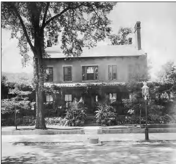
The superintendent's quarters (USMA Library)
